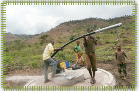
Final stages in constructing the Mshkamaro Shallow Well.
