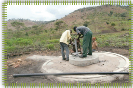
Final stages in constructing the Mshkamaro Shallow Well.
